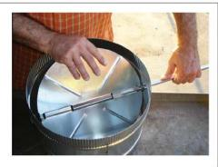
3. Spotweld or rivet the regulator in place, making sure the handle and blade are in corresponding positions.
