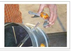
4. Center the blade and secure the system with a self-drilling screw.
